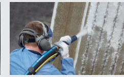
150 psi: Abrasive blasting
