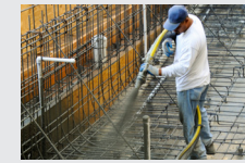
180 psi: Shotcrete applications
